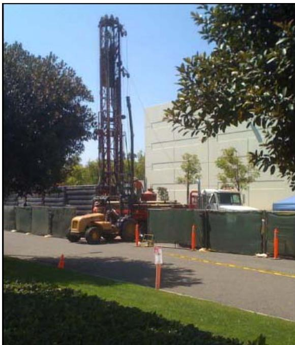
*Pictured above is a drill rig constructing a groundwater monitoring well west of the Site.*
